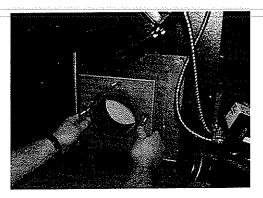
6- Remove with caution the combustion chamber with its support and put it down on a safe surface.
