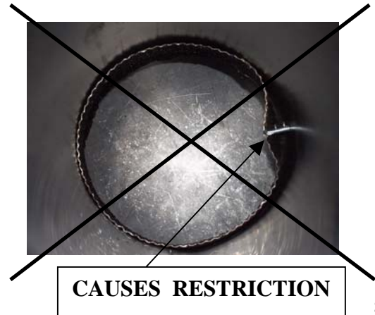
FAULTY INSTALLATION
