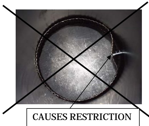
IMPROPER INSTALLATION
